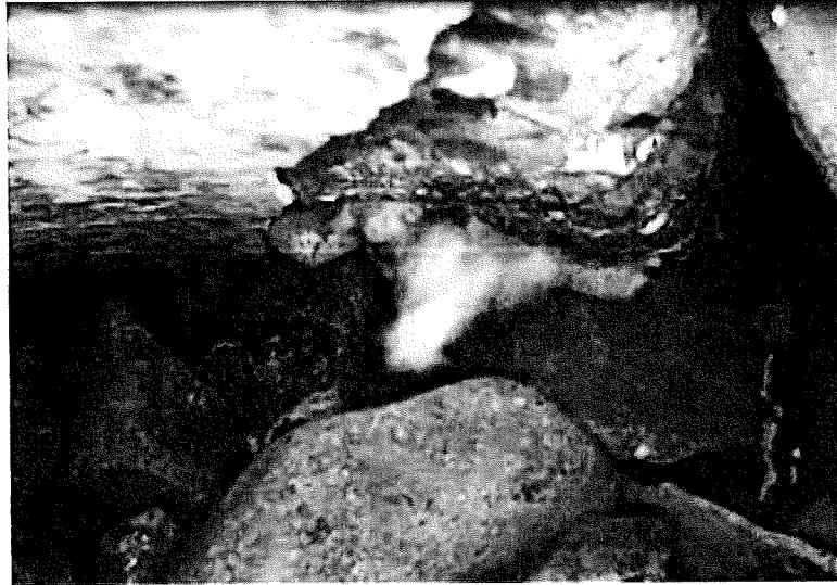
Figure 1.1 12-Inch River Street Siphon Cobble
