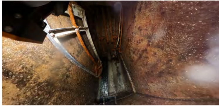
Figure 2.1 Jefferson Avenue Control Structure
