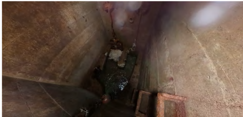
Figure 1.2 River Street Control Structure
