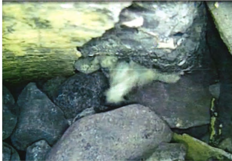
Figure 1.1 12-Inch River Street Siphon Cobble
